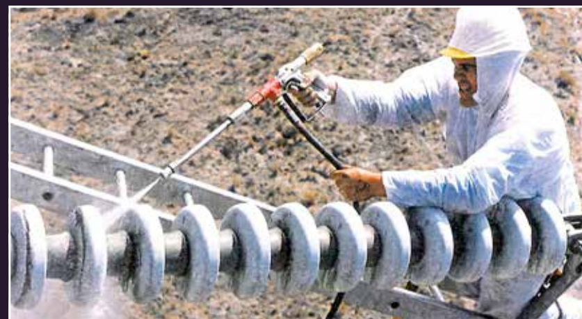
Ash is cleaned from a 220 kV strain insulator string using pressurised water following the 1995 Ruapehu eruption, New Zealand (Transpower New Zealand)
